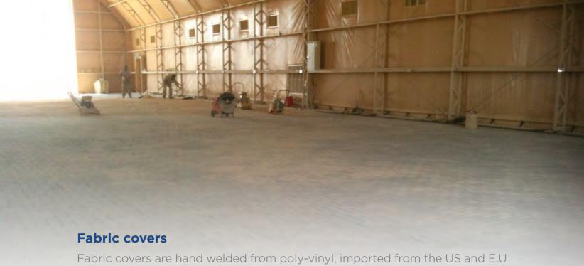
Fabric covers are hand welded from poly-vinyl, imported from the US and E.U in rolls. The material is fire proof, water proof, mildew resistant, UV proof and cooperates an inherent blackout material. Material is individually measured, cut and welded to fit steel frames.
